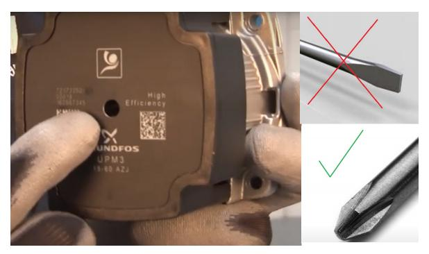
Following a prolonged period of not being used such as in the summer, a number of pumps may not run when being turned on for the first time. This is usually due to a build up of debris in the pump which will prevent the internal rotor from turning.
